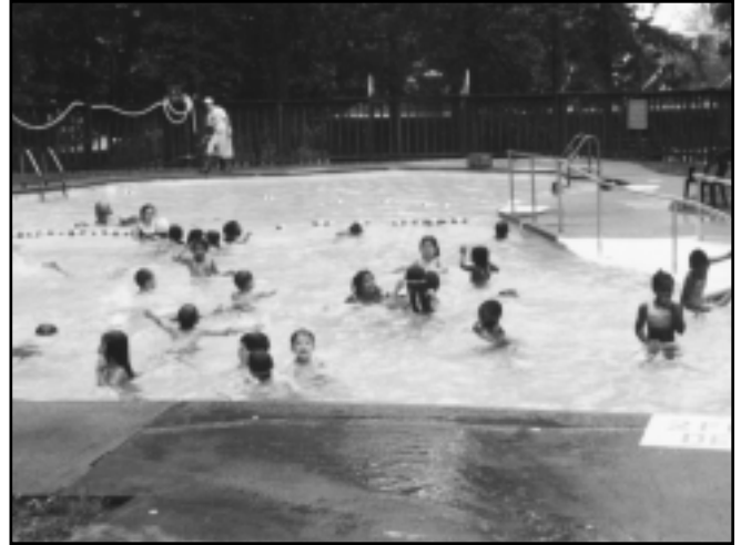
This Wagon Road Camp pool will be renovated right after summer camp, and will be joined by a new pool that will greatly expand Wagon Road's cooling capacity.
